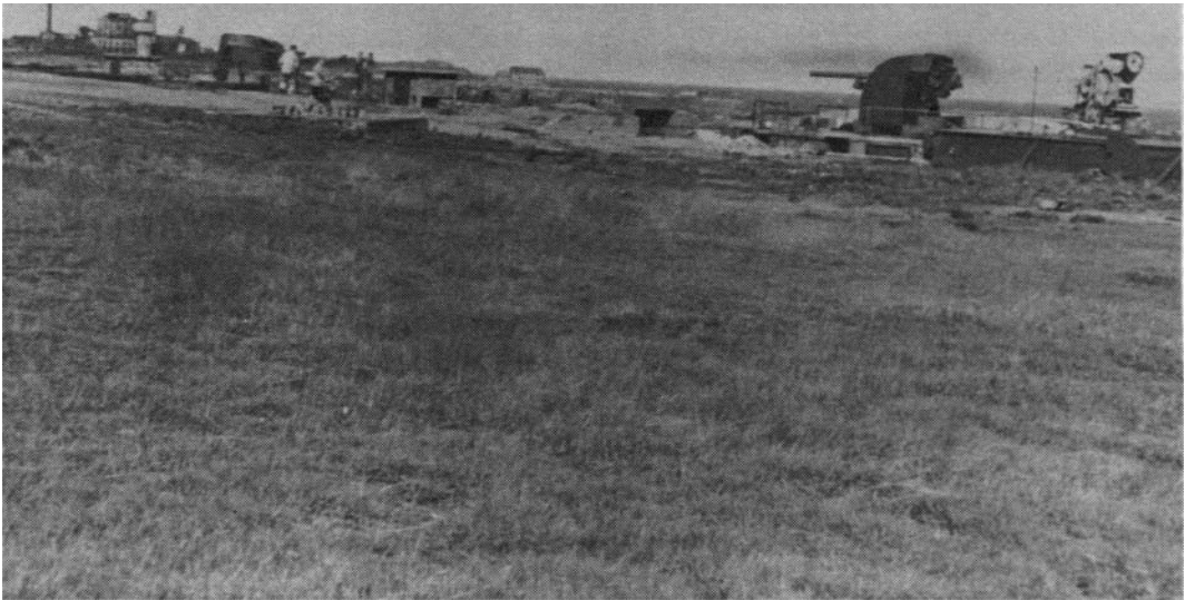
Figure 1: Chapel Battery, Sydney, N.S. View of both guns showing twin four-inch barrels.
