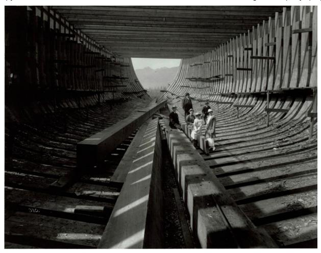
**Image 1:** A group including Andy Wallace, Mrs. H.W. Brown, and Mrs. Geraldine Wolvin sit for the photographer in the framed hull of the *Mabel Brown* at Wallace Shipyards Ltd., North Vancouver on 9 July 1916. Note the size of first-growth timber required for the construction of these vessels." Photo from Vancouver Public Library photo, #20058.
