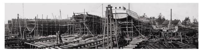
**Image 3:** *Malahat* building on Cameron-Genoa Mills Shipbuilding ways, 1917. What is probably the *Jean Steedman* and two of four wood cargo steamers also built by the company in the midst of construction lie off to the left. Photo courtesy of Ronald Greene, Capital Iron collection, Victoria.
