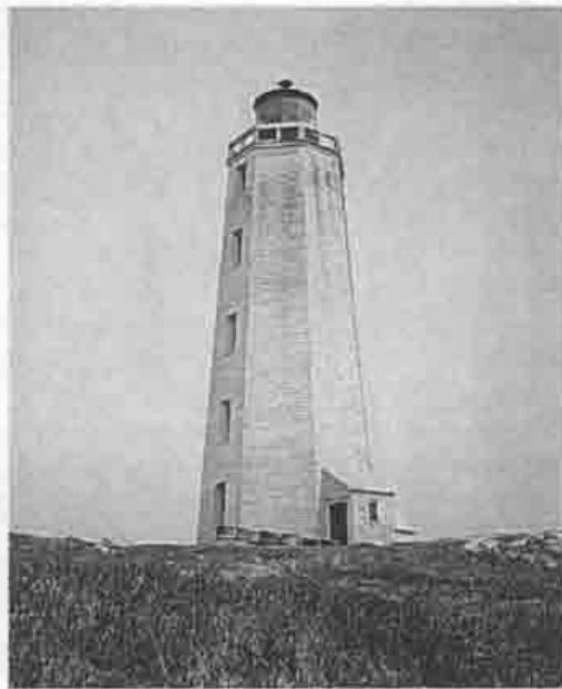
The original 92-foot octagonal Cape Roseway lighthouse, constructed of locally cut stone in 1788, is shown here as it appeared to us in 1952. Seven years later it was struck by lightning. The ensuing fire destroyed its heavy oak supporting timbers resulting in its replacement with a 48-foot concrete tower.
