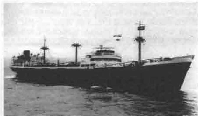
Fig. 3: Bulk carrier Photinia (Stag Line Ltd.); G.T. 7660; length, 479.7 ft., beam, 60.25 ft.; single screw diesel, six cargo holds.
