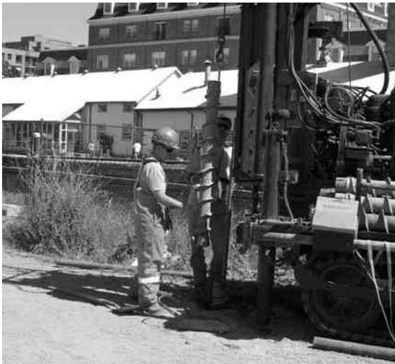
Boreholes were drilled to determine the character of the soil on each side of the dock. This is being done to ensure the ship in the dock dry for a protracted period of time and visitors will be safe.
