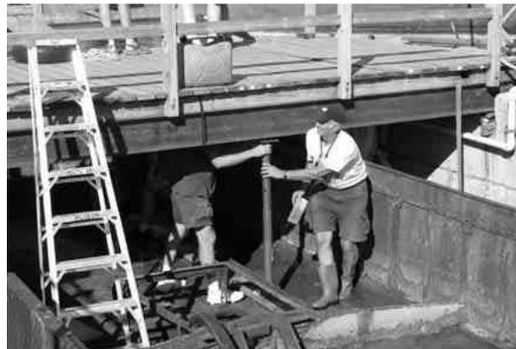
Once the ship was in, the dock the 'gate' had to be drawn across the entrance to give further protection to the *Alexander Henry*. This was done to minimize strain on the mooring lines keeping the ship in place. An open dock in a heavy fall southerly has the characteristic of a wave chamber.
